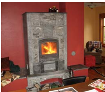
Figure 2. Photograph of Barkman family contraflow masonry heater. Pleasant Hill, Oregon.
